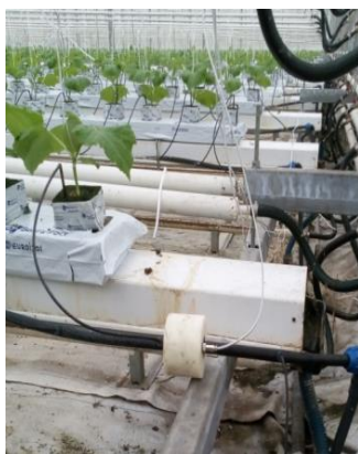
Fig. 1. Acoustic-magnetic device installed in the hydroponic solution supply system
